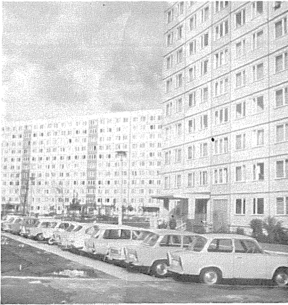
Berlin, DDR: Blocks of flats in the P2 type industrialised building system, factories close to homes, private cars parked in the open, but carefully wrapped against weather and vandals.
